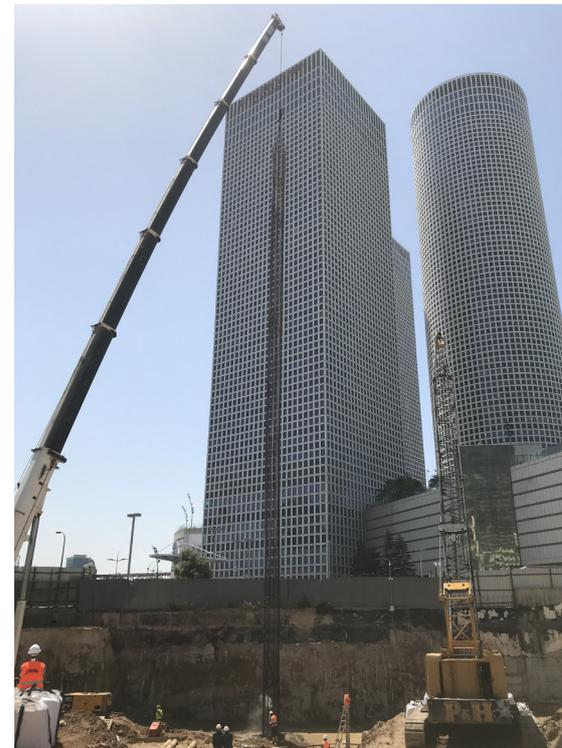
Pile reinforcement installation with O-cell assembly.
